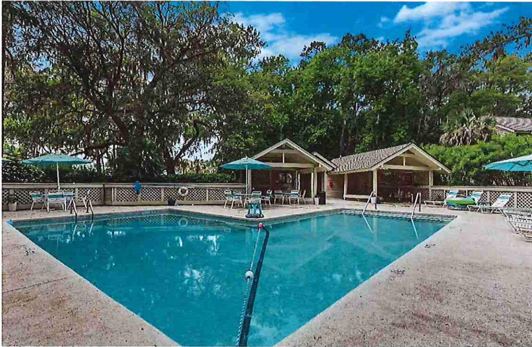
Before Picture of the Pool Deck
